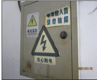
Photo of the inside of the main production hall Electric shock warning.JPG
